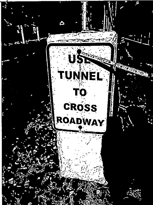
PHOTO 18 DESCRIPTION SOUTHEAST PEDESTRIAN CROSSING SIGN. CORRODED BOLTS TOP & BOTTOM
