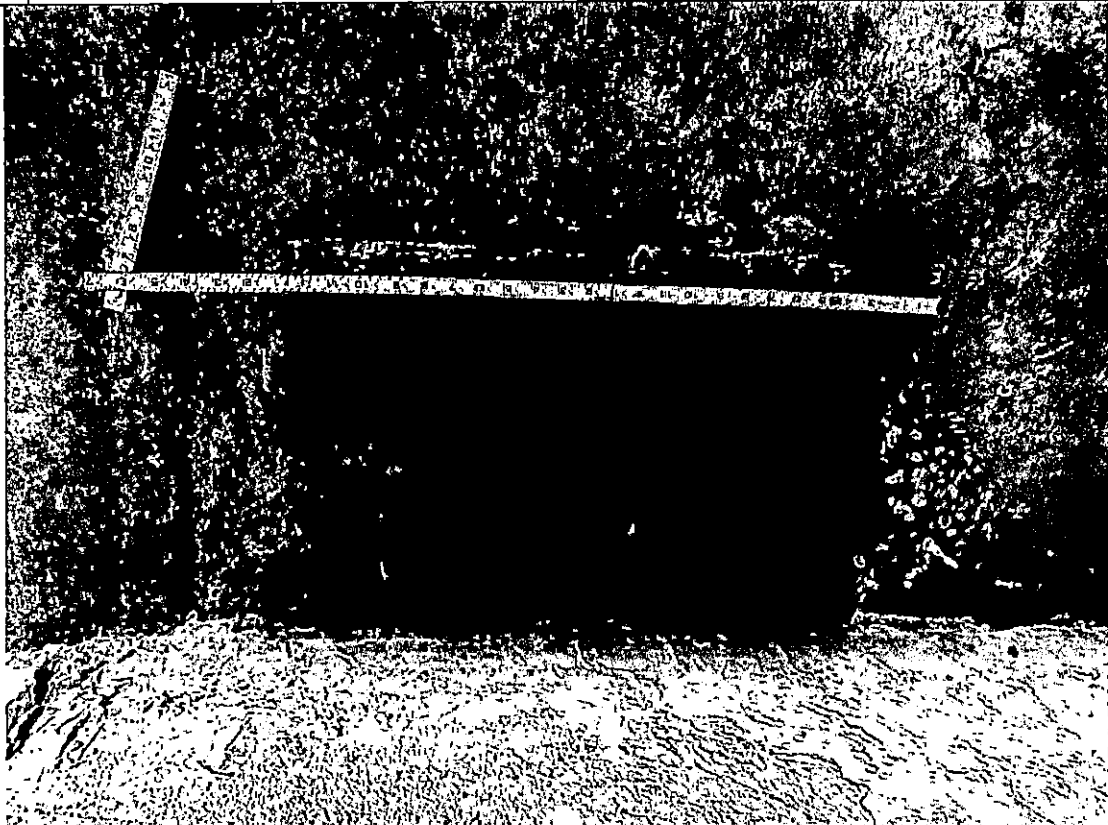
PHOTO 24 DESCRIPTION 2"x5"x1" DEEP SPALL NEAR DRAINAGE INLET
