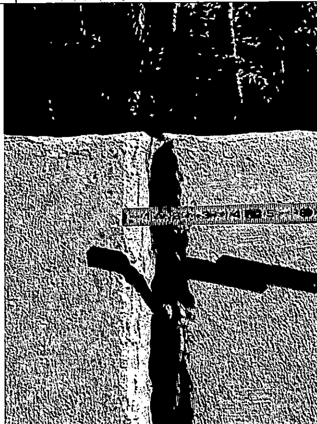
PHOTO 44 DESCRIPTION 2" JOINT IN RETAINING WALL (TYPICAL)
