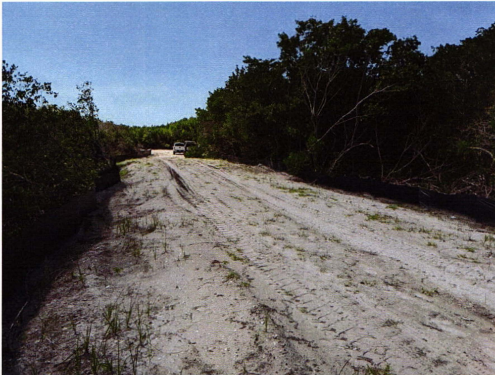
Photo #8 – Temporary repair haul road looking South.
