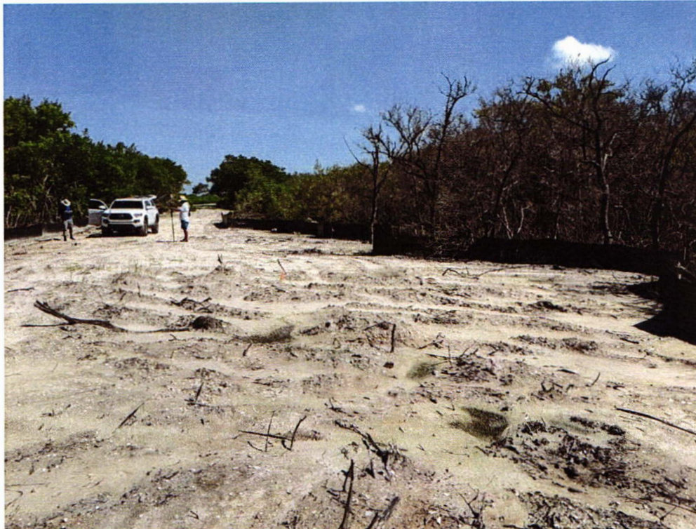
Photo #6 – Southern limits of temporary haul road looking North.
