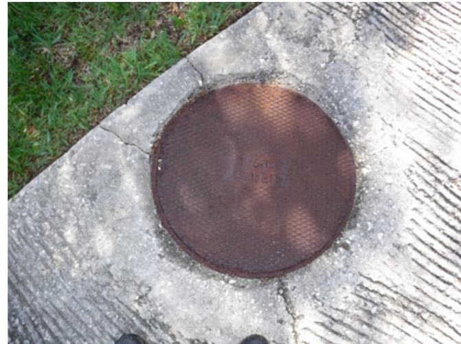
Cracks adjacent to manholes may contribute to infiltration of saltwater into utility conveyance systems in areas of regular tidal flooding.
