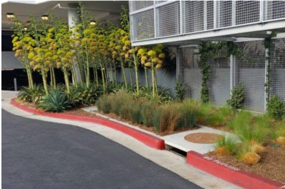
Figure 5: Installed Modular / Linear Wetland System
