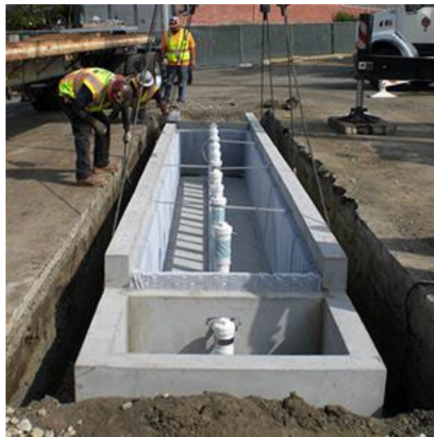
Figure 6: Installation of Modular / Linear Wetland System
