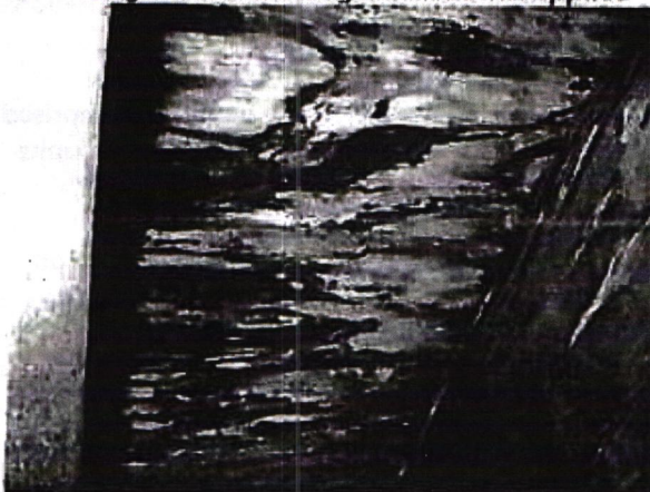
003 - Rotten wood sheathing and joist @ roof
