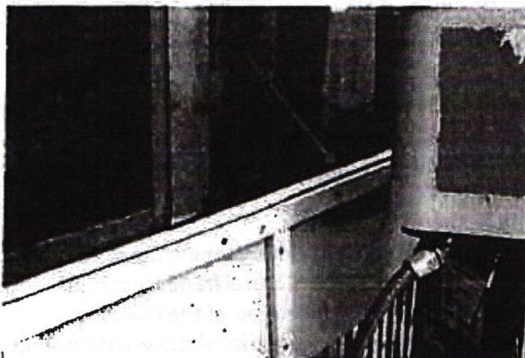
023 - Bowed window sill flashing, no sealant
