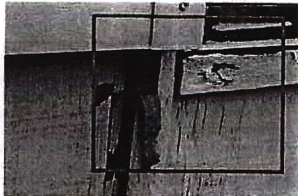
020 - Rotten wood siding beneath window
