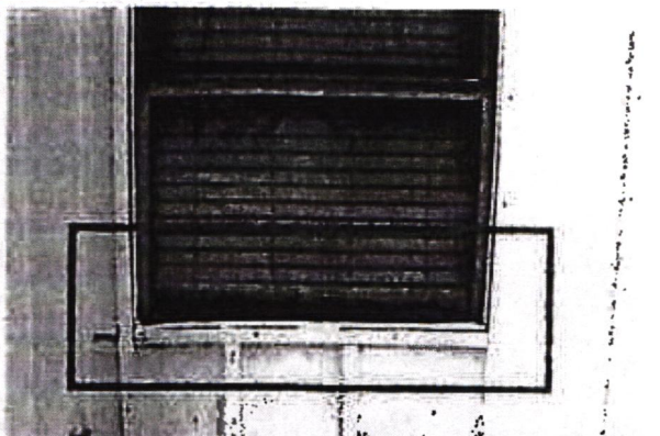
012 - Bowed framing and window caused by settling of framing members
