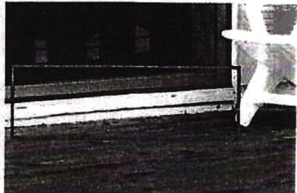
022 - Rusty fasteners and no sealant a sliding glass frame sill
