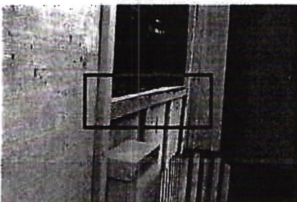
017 - Bowed window sill flashing, no sealant
