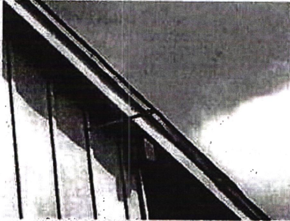
001 - Original roof flashing bent and mis-applied
