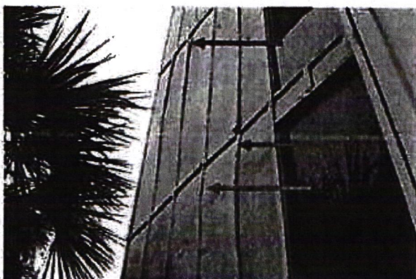
016 - Bowed exterior sheathing and loose battens
