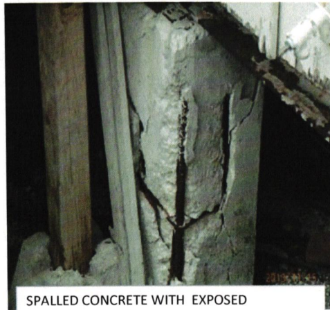
SPALLED CONCRETE WITH EXPOSED REINFORCEMENT .
