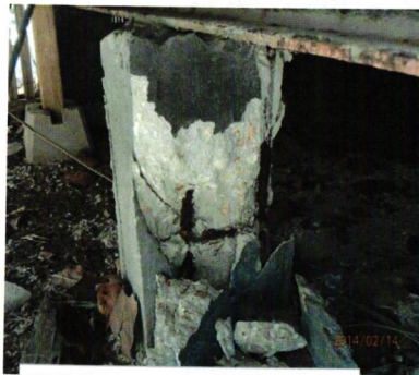
SPALLED CONCRETE WITH EXPOSED REINFORCEMENT
