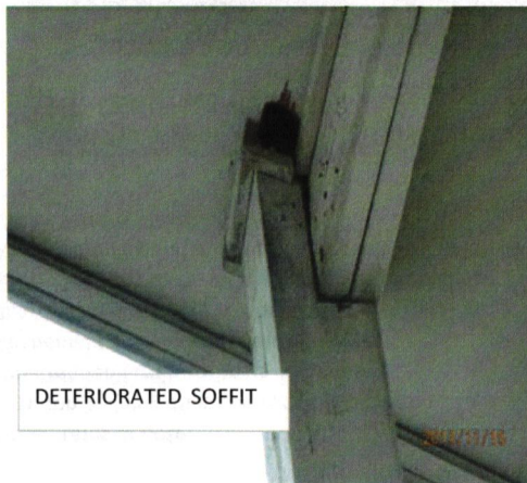
FLOOR FALLING . NO LONGER SUPPORTING POST ABOVE
