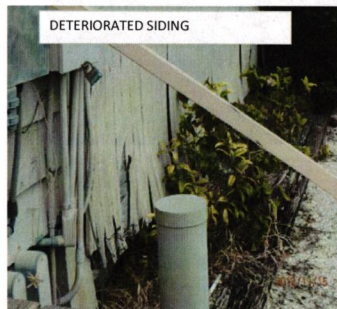
DETERIORATED SIDING
