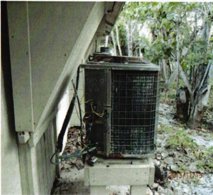
DETERIORATION OF METAL AT MULTIPLE AREAS OF AN AIR CONDITIONIN UNIT.
