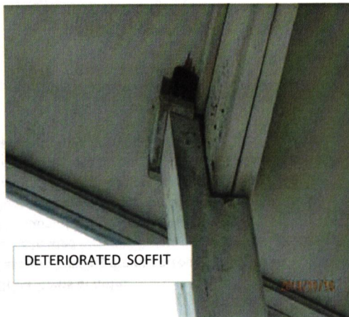
FLOOR FALLING . NO LONGER SUPPORTING POST ABOVE
