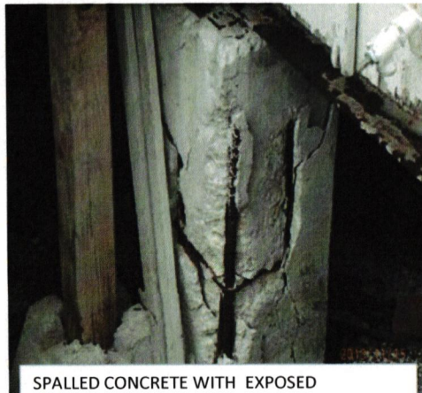
SPALLED CONCRETE WITH EXPOSED REINFORCEMENT .
