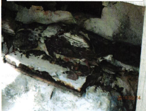
DETERIORATION IN BEAM , WELD AND WELD PLATE
