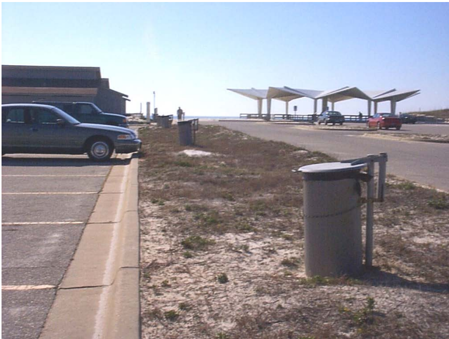
Example of trash receptacle anchored into the ground so it is not easily turned over.
