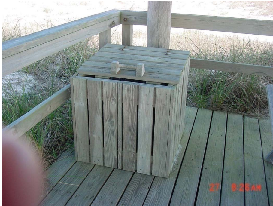
Example of predator proof trash receptacle at Perdido Key State Park. Metal trash can is stored inside. Cover must be tight fitting and made of material heavy enough to stop animals such as raccoons.
