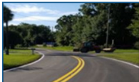
Repaved road in Pasco County, FL
