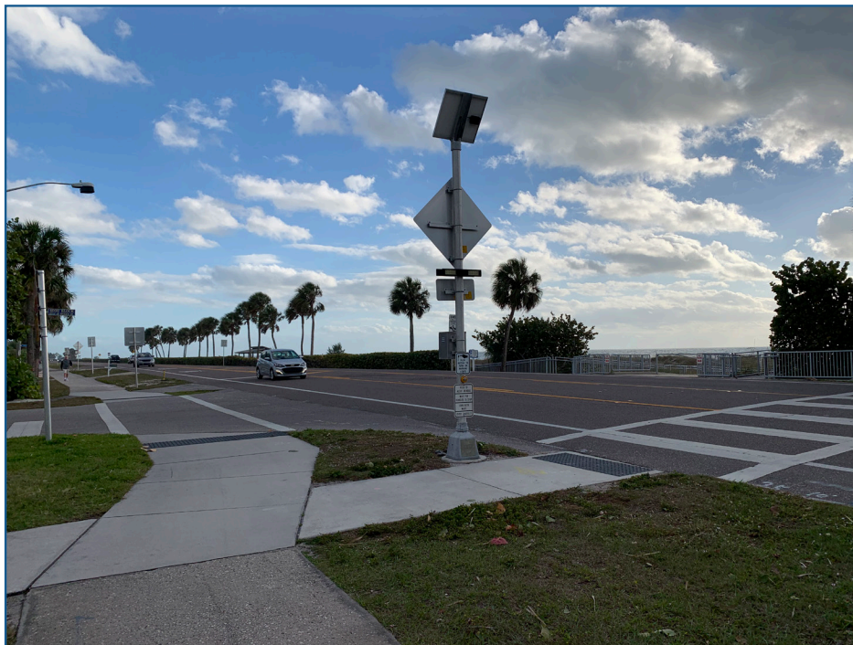
Figure 12: Rectangular Rapid Flashing Beacon near Bayfront Park
