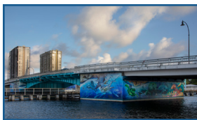
Bascule Bridge Improvements, Pompano Beach, FL
