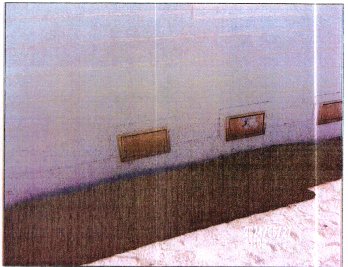
Photo Six Caption: Flood Vent in Garage– Outside View
