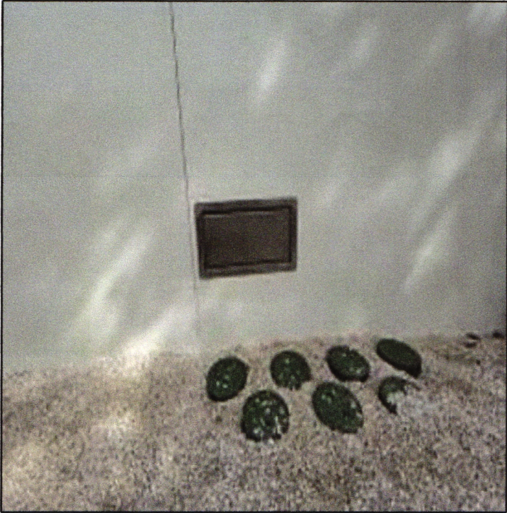
VENT PHOTO TAKEN ON JANUARY 22, 2024
