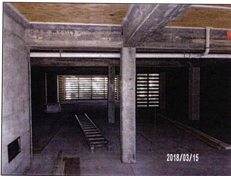
PHOTO FIVE CAPTION: 1"x8" SLAT WALLS WITH 3/4" GAPS (INSIDE VIEW)
