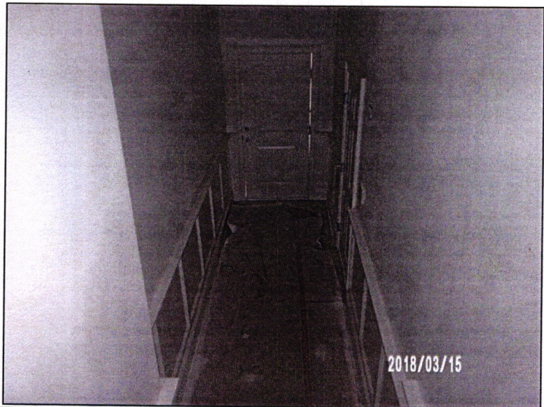
PHOTO FIVE CAPTION: VESTIBULE FROM TOP OF STAIRS
