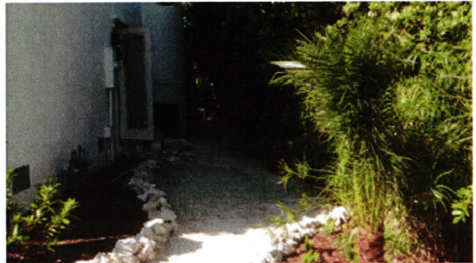
NORTH SIDE WITH VENTS:
