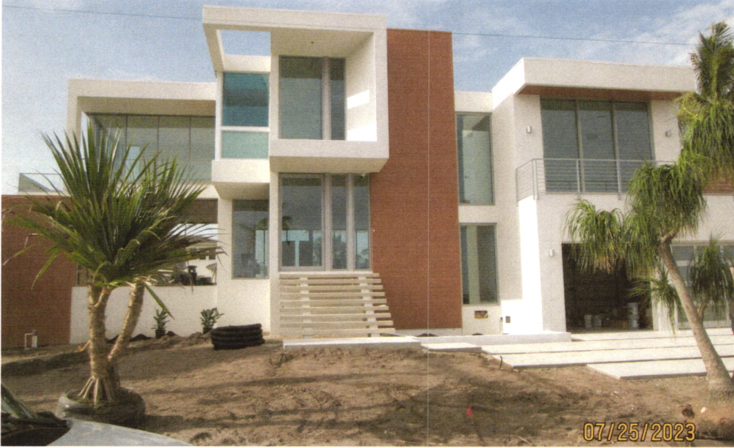
Photo One Caption: FRONT VIEW (NORTH SIDE)
