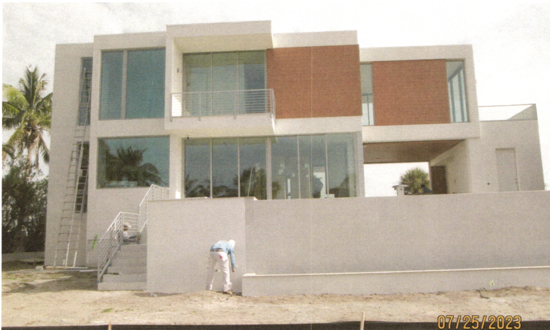
Photo Two Caption: REAR VIEW (SOUTH SIDE)
