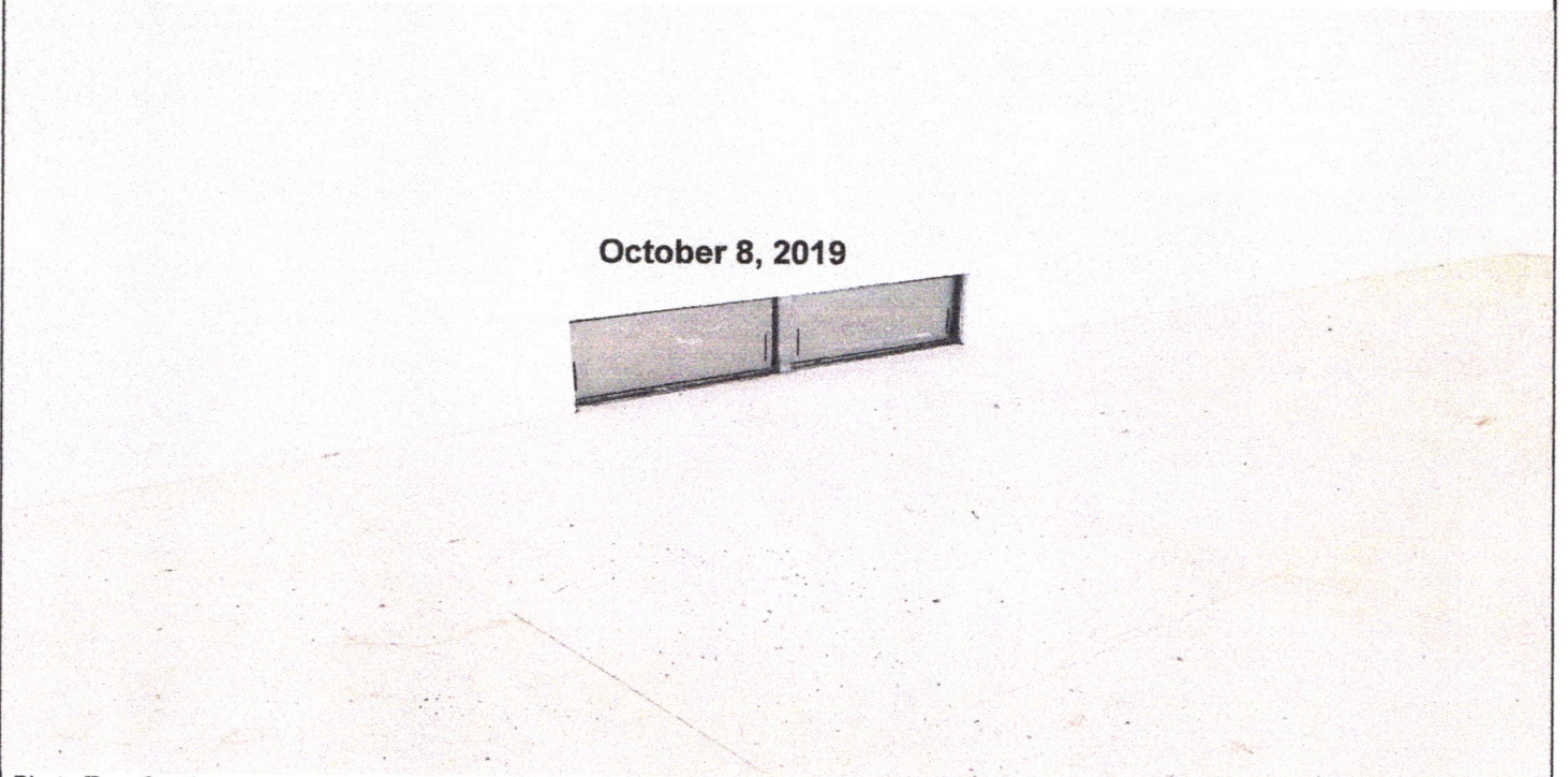
Photo Two Caption Vent Photo
