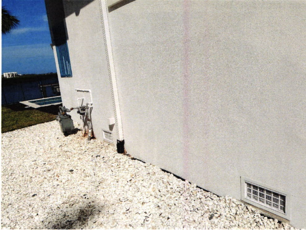
(11/14/2024) 2 Flood Vents on Left Rear Wall of Garage Area.
