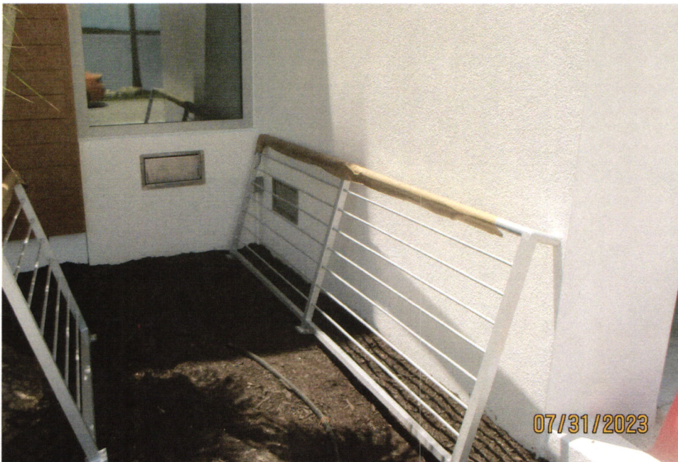
Photo Four Caption: TYPICAL FLOW-THRU VENTS
