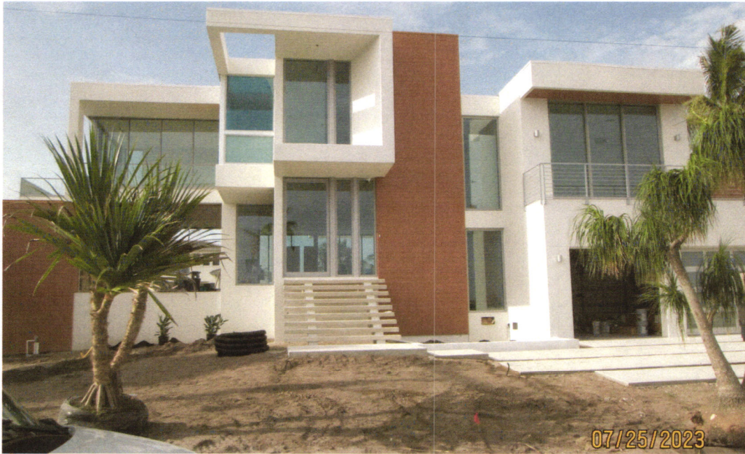
Photo One Caption: FRONT VIEW (NORTH SIDE)
