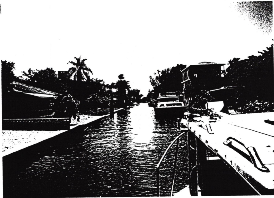
Canal 17 (between Jungle Queen Way and Tarawitt Drive) is typical of Canals 17 through 19. The canals are narrow (less than 40 feet between the seawalls) and are shallow. The canal contains several seawalls that have failed due to lack of sufficient toe penetration. Canal 18 also contains one stand of mangroves which is encroaching into the canal. The narrow width of these canals may preclude further dredging.
