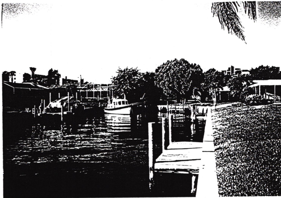
Canal 38 (between Birdie Lane and Putting Green Lane) shows evidence of seawall failure with the installation of wood piles at the face of the wall to prevent toe or tieback failure.
