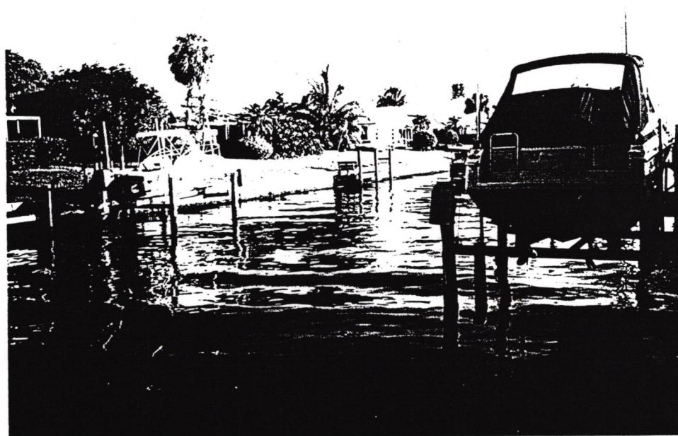
Canal 36 (between Chipping Lane and Wedge Lane) is typical of the canals in Country Club Shores. The canals are wide with concrete seawalls. Most of the homes along the canal have marginal docks, many with boat lifts. The seawall in the photograph shows evidence of tieback replacement which is common in Country Club shores.
