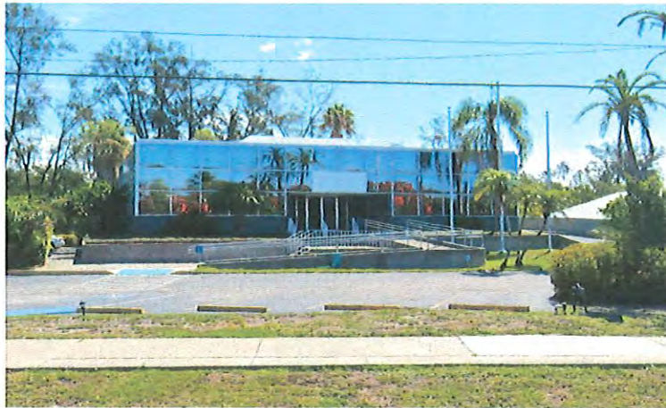
Existing Abandoned Former Bank Building (to be demolished)
