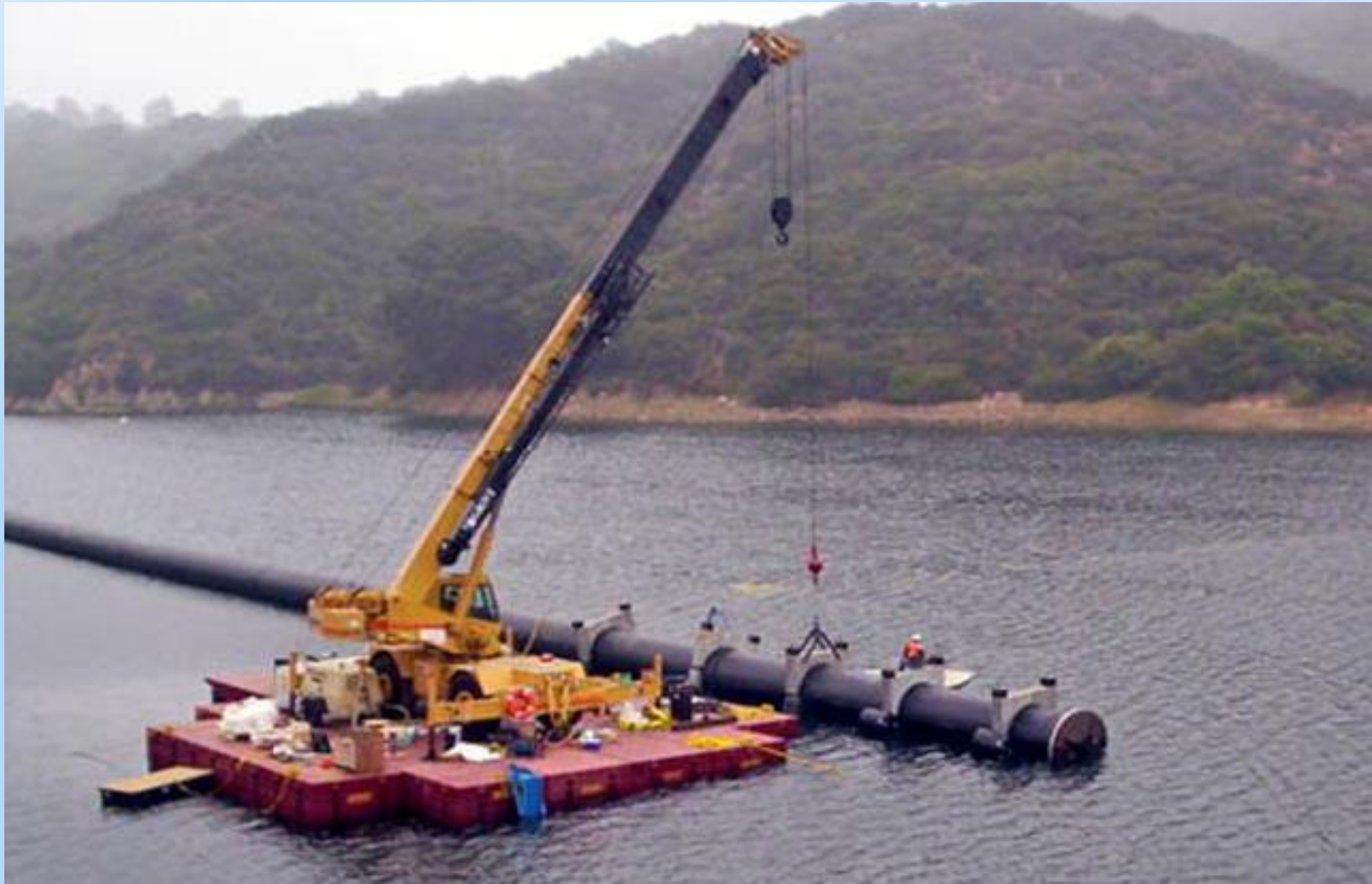
Subaqueous Pipe Installation
