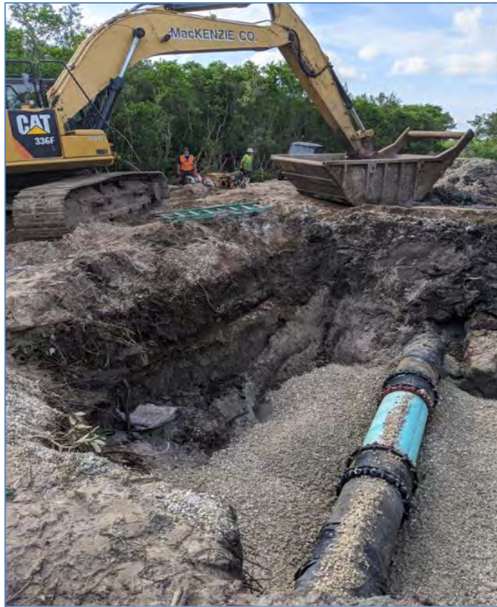
Figure 1-1 Repair of Existing Force Main Within Mangroves
